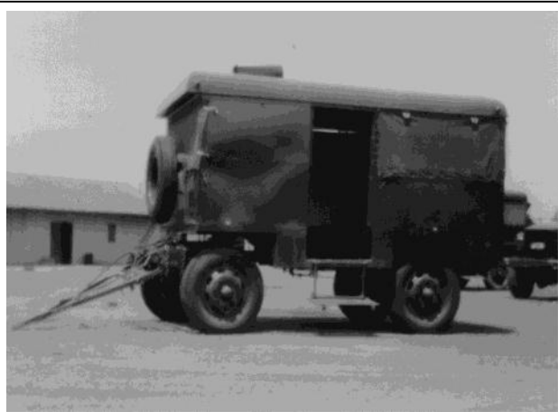
Left: A late 1950s production 4-wheel Wiles Cooker, finished in gloss Deep Bronze Green. The main difference was the running gear manufactured by Freighters, and fitted with 20-inch wheel assemblies. (D McCallum)
